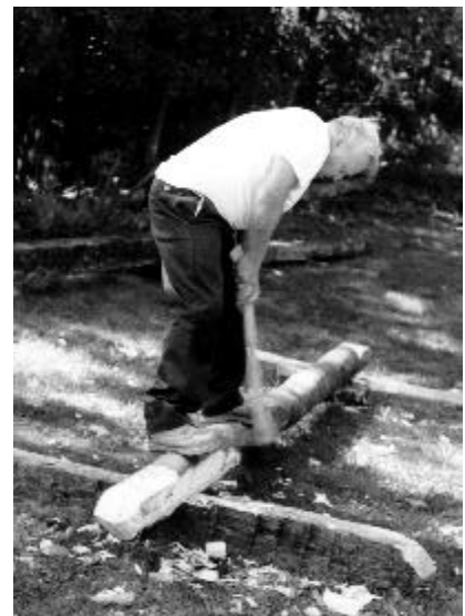
Dick Babcock demonstrates beam-hewing at the HMF Fall Festival
