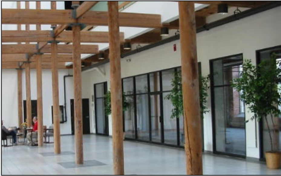
Adams Mill – vacant commercial floor
