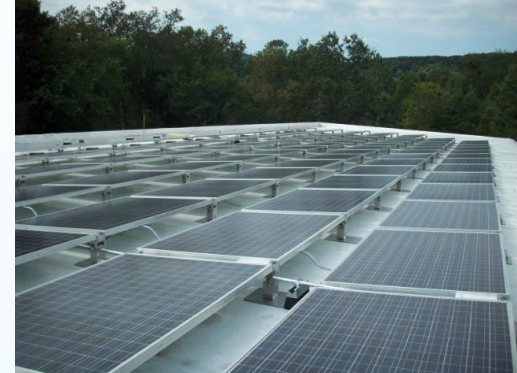
William's Library Shelving Facility
